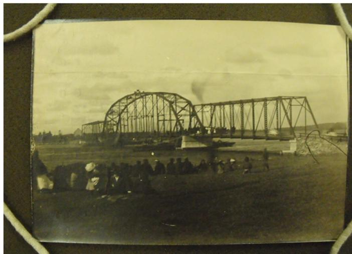
FIGURE 2. The central section of the Indian Sluice Bridge being floated into place, 1909.
