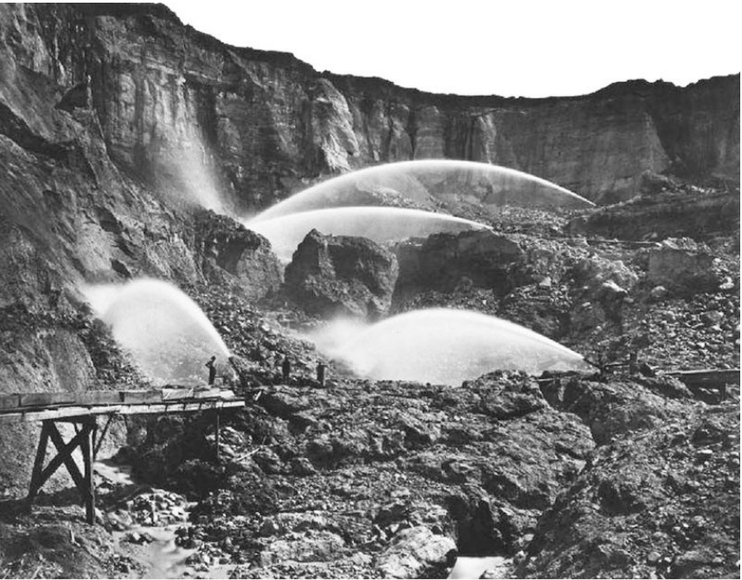
FIGURE 1. Four hydraulic monitors at work processing Tertiary gravels at Malakoff Diggins.
