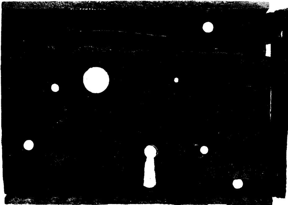
23 Iron-rim lock. Forged three-bolt Carpenter-type lock. The latch is a pivoting bar with its head permanently projecting outside the case. The head is bevelled so that it rises as it passes a catch on the door frame. *Photo by R. Chan.*
