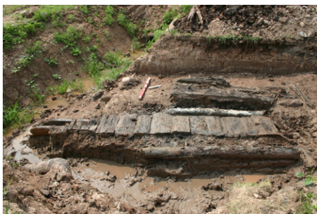
Culvert, possibly from 17th-century road construction through dyked marsh land at Grand-Pré. Photo by Rob Ferguson, Parks Canada.
