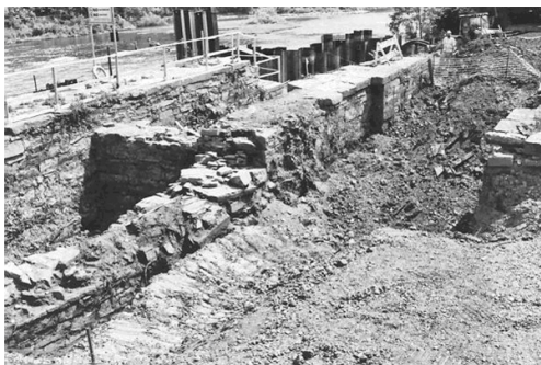
Riverside wall of Guard Lock showing lower upstream extension; dam abutment in background. View south.
