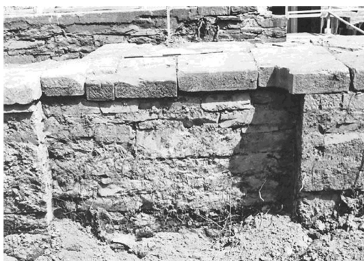
Upstream mitre gate recess of Guard Lock wall on river side. View southeast.
