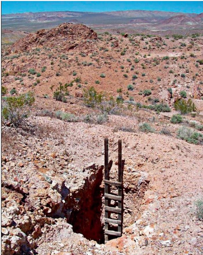
FIGURE 3. Unsupported shaft collar. (Photo courtesy of Sterling White, BLM.)
