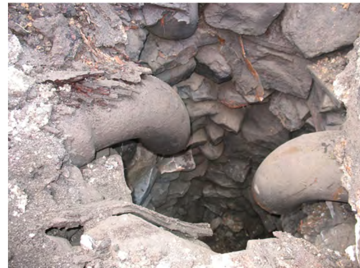
FIGURE 3. One of six stone-lined cesspits with drain pipes.
