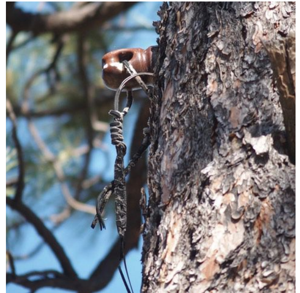
FIGURE 6. Tree-mounted, brown-glazed, lag-screw porcelain insulator with tie wire and drop wire of a possible U.S. Army Military Police Corps telephone line of Project Y vintage. (Photo courtesy of Schön Levy.)
