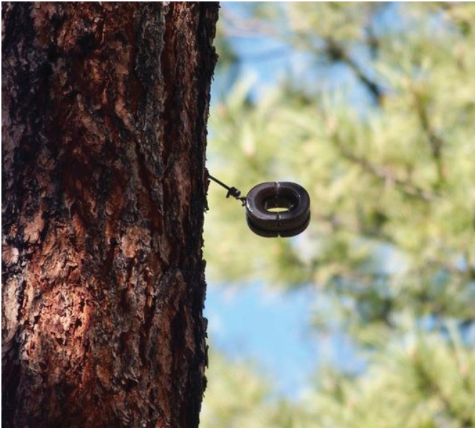
FIGURE 5. Tree-mounted, brown-glazed, split-knob porcelain insulator of the ca. 1937 USFS telephone line. (Photo courtesy of Schön Levy.)
