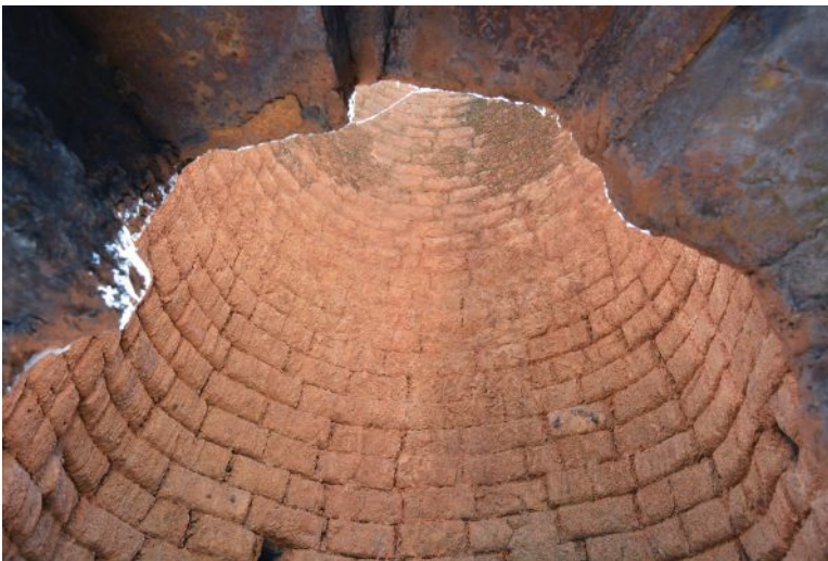
FIGURE 4 (left). Interior brickwork of kiln stacks. (Photo courtesy of the author.)
